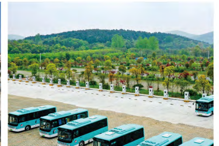
Zipeng mountain public bus EV charging station in Hefei, China 🇨🇳
