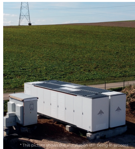
Two Sungrow PowerTitan ST2752UX storage systems and just one SC3125HV-30 inverter are installed in one section of the solar park
