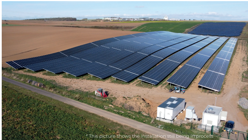
Two Sungrow PowerTitan ST2752UX storage systems and just one SC3125HV-30 inverter are installed in one section of the solar park
